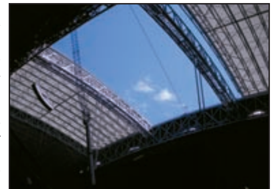
Powered by 128 motors, the retractable roof can be opened or closed in nine minutes. On a clear day, it is visible five miles above the stadium.
