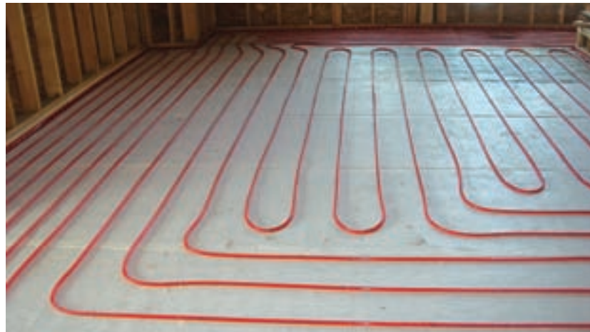
Each of three buildings at Spring Creek residential community incorporates low-temperature radiant heating via 550,000 feet of RAUPEX, and geothermal systems from Geo Furnace Technologies as its main source of heat.
