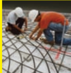
Slab on Grade
