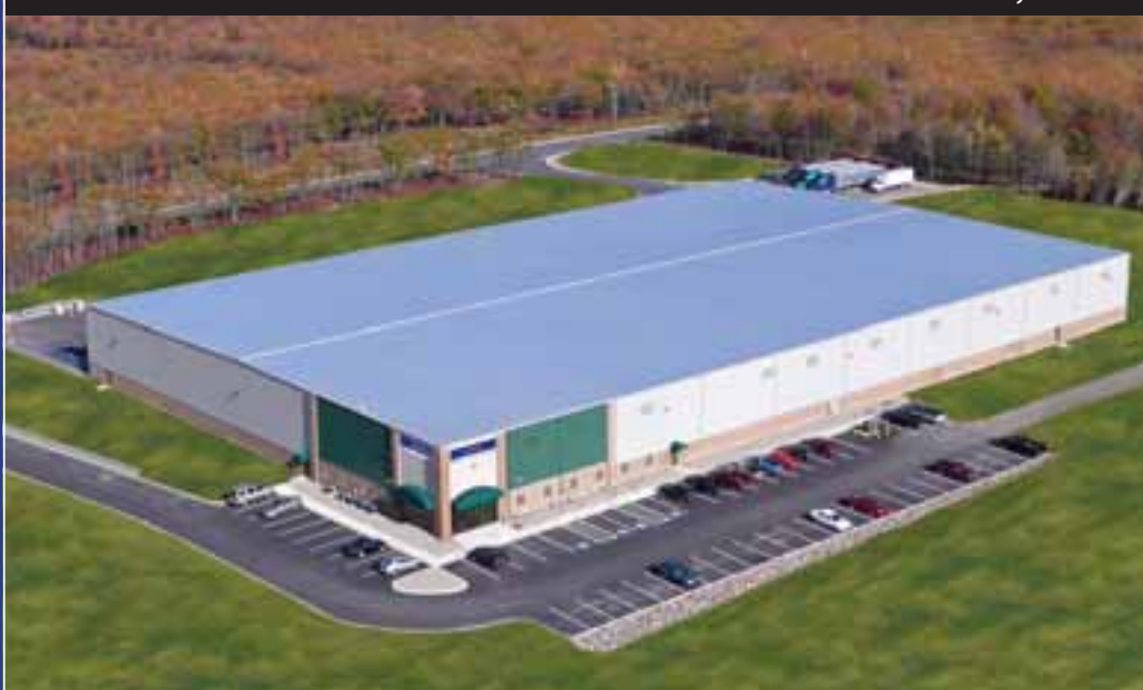
JONES STEPHENS CORP. NORTH - POTTSVILLE, PA
