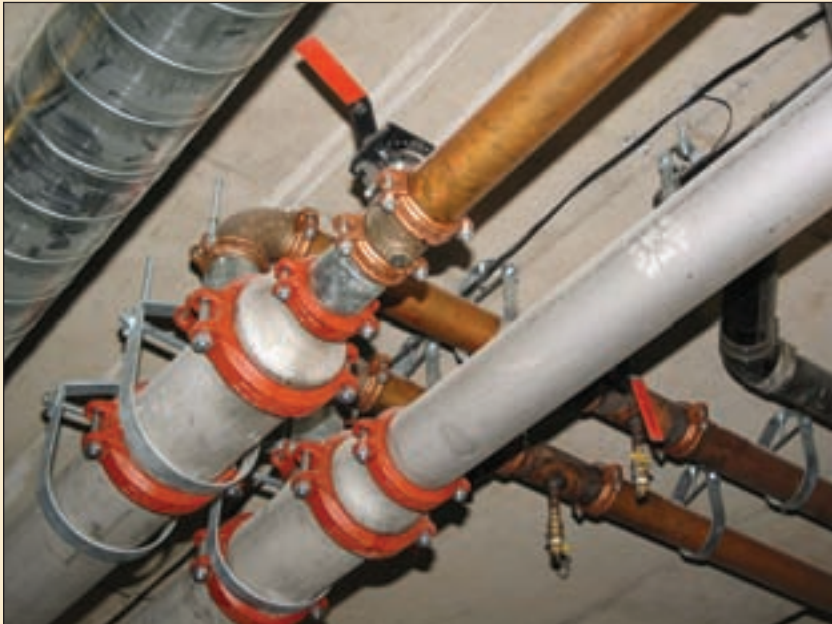
Grooved piping systems have a union at every joint for easy re-routing during system expansion.
