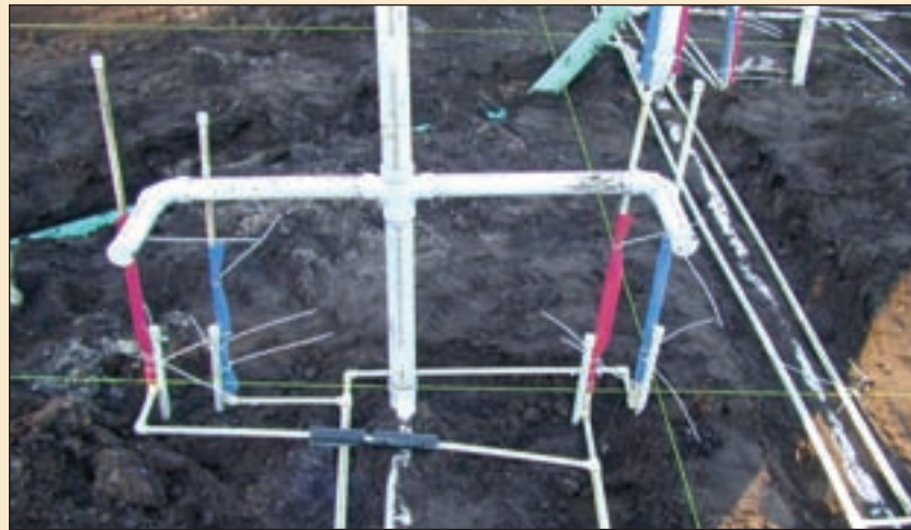
The combined benefits of durable CPVC pipe and fittings make such systems an ideal choice for joints underslab installation.
