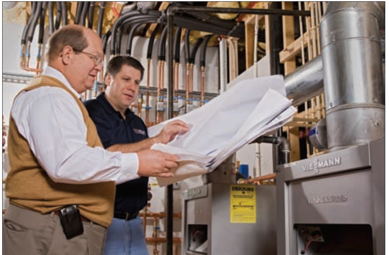
Gary "Skipper" Joyce (l), owner of manufacturers rep, the Joyce Agency, reviews mechanical room plans with Dan Foley.
